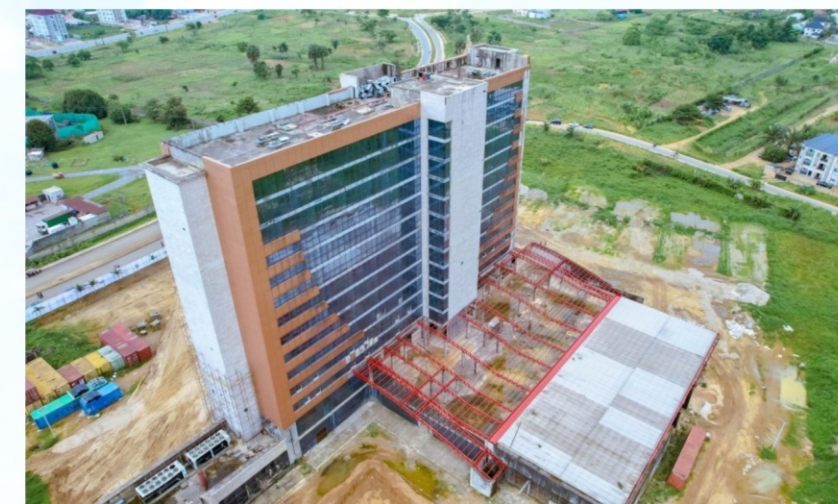
▲ Ongoing Ibom International Hotel, Uyo
