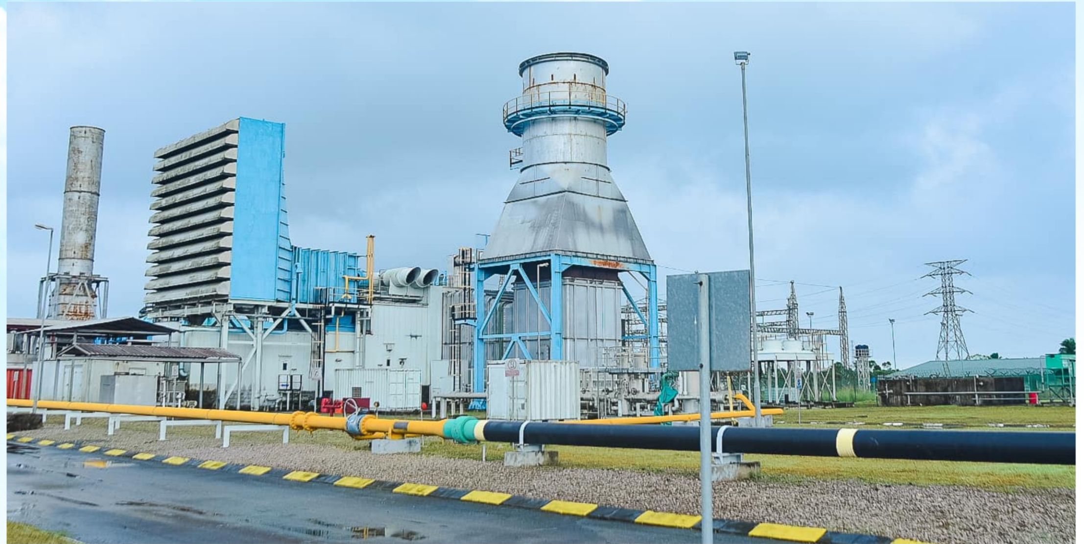
▲ Ibom Power Plant
